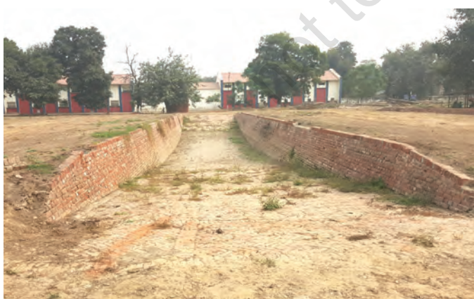
Fig. 1.9(a): Structure of bunker-type silo
