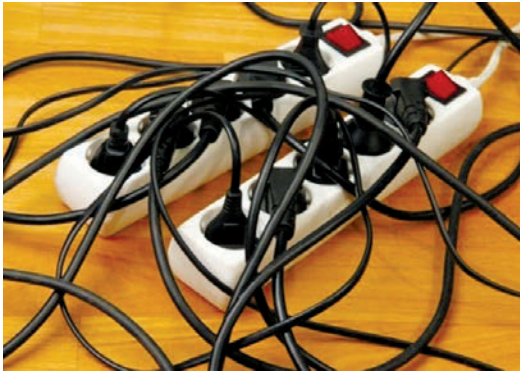
Fig. 1.29: Overloaded extension cords
