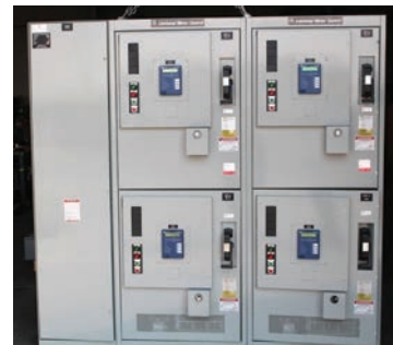
Fig. 8.13 Multi-door control panel
