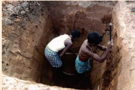
Fig.1 Making a pit for earthing
