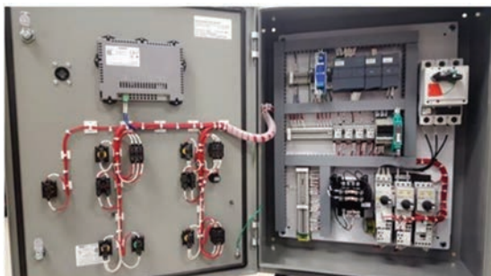
Fig. 8.12 One-door control panel
