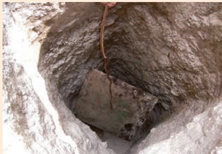
Fig. 2 Copper plate set in the pit
