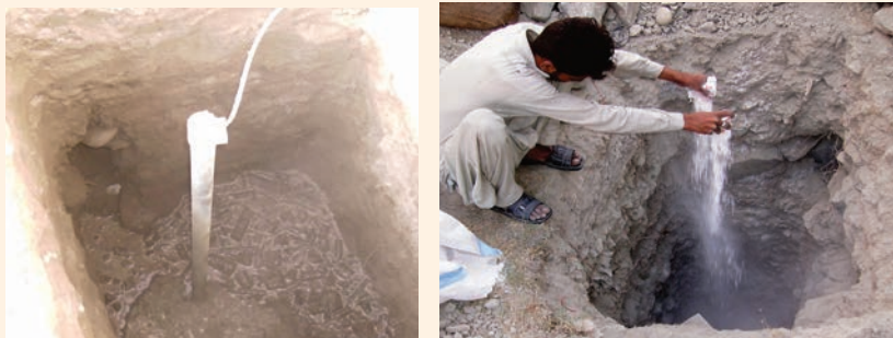
Fig. 4 Pit filled with mud, sand and stones
