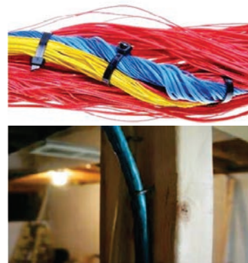
Fig. 9.75 Securing of cables
