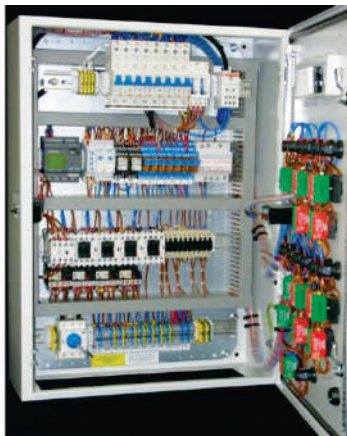
Fig. 8.16(a) Correct raceway (routing) of cable
