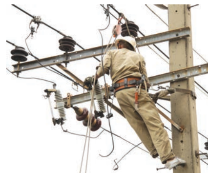
Fig.1.1(b) A lineman repairing electric fault
