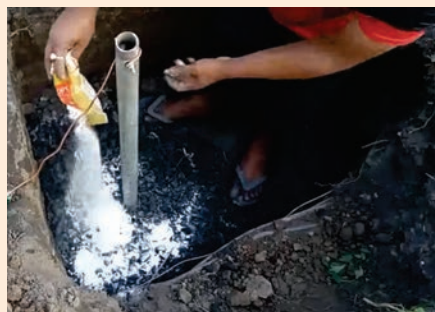
Fig. 3 Copper plate and surface are connected with a pipe
